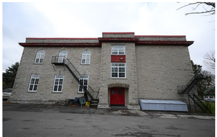
Fig. 4 Church Street School Apartments northeast façade, Credit: Tim Austen Photos, 2025
