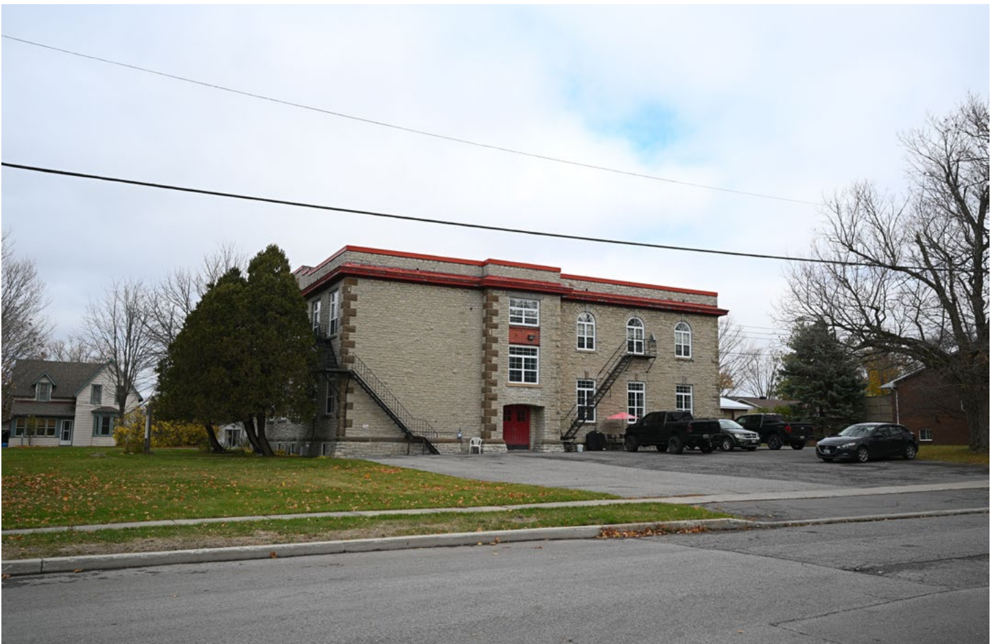
Fig. 5 Church Street School Apartments William Street façade, Credit: Tim Austen Photos, 2025
