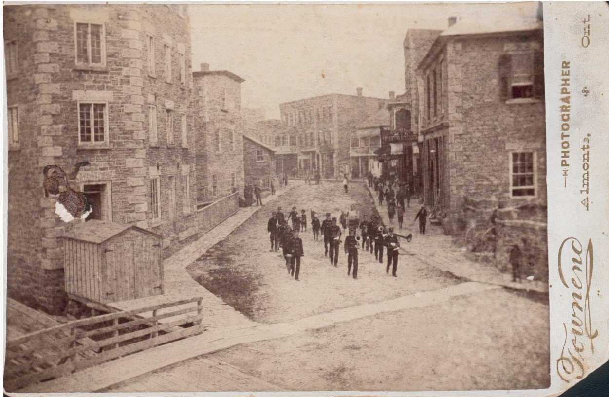
Caption: This photograph from the late 19th century shows the varied rooflines constructed as part of Mill Street's initial development.
