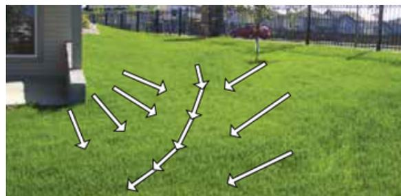
Internal drainage swales (above and below).
