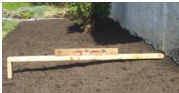
*Dirt or sod should slope down from the wall on a continuous angle.*
