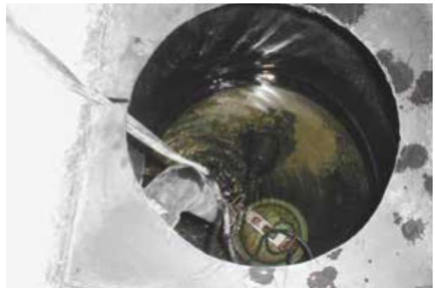
*A sump pit with submersible sump pump.*
