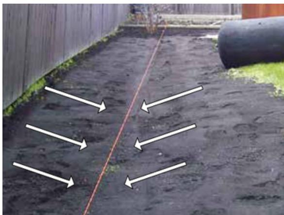
A swale should slope to channel water away from the home.
