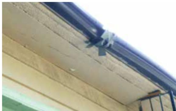
**Replace eavestroughs that have holes or cracks.**
