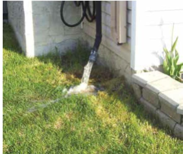
*Incorrect placement of splash pad. Splash pad is missing and downspout is not long enough.*
