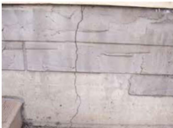
**Crack in the foundation wall of a home.**
