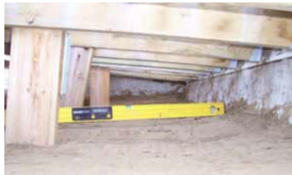
**Under steps and decks can be weak spots in lot grading.**
