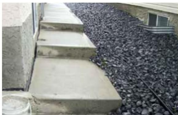
**When lot grading, it's important to check the slope from the basement wall.**
