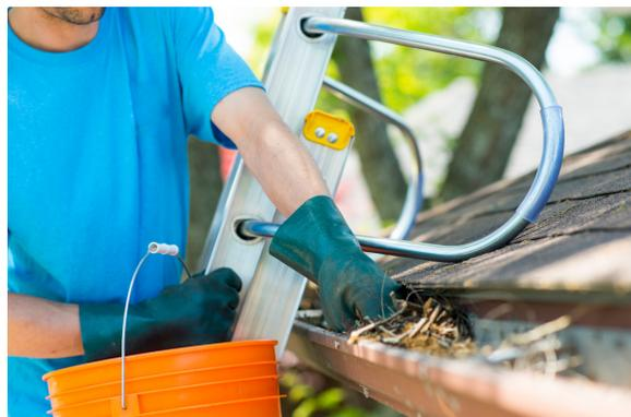
**Eavestroughs should be cleaned regularly of leaves and debris.**
