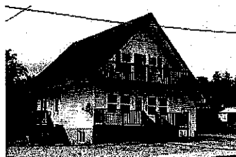
Example of post-modern style, on Queen Street.
