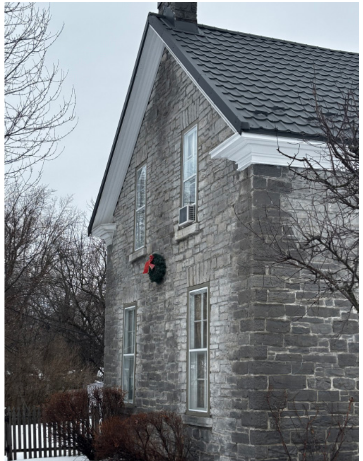
Fig. 7 Snedden House rectangular windows and returned eaves, Credit: The Municipality of Mississippi Mills
