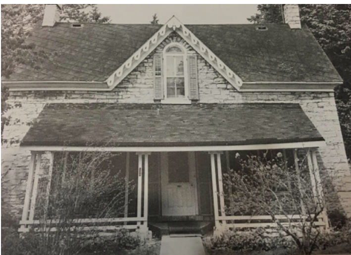
Fig. 4 Snedden House before removal of a later veranda, not the original, Credit: Tales of Almonte Facebook page, October 2018
