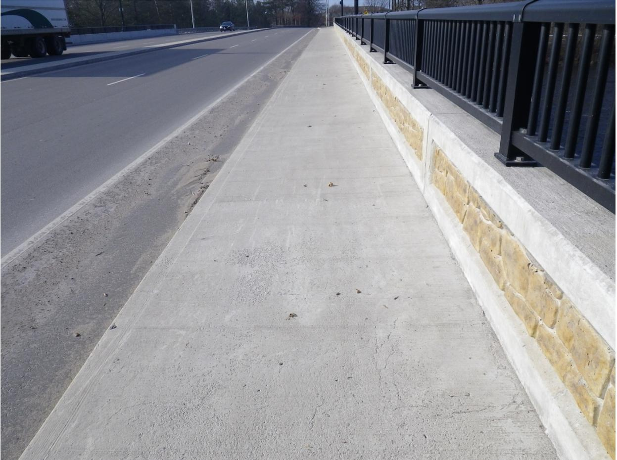
Option 3 - Concrete parapet with decorative finish and steel railing
