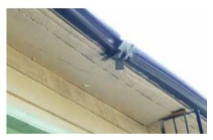
Replace eavestroughs that have holes or cracks.
