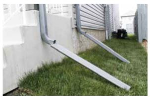
Downspouts take water away from eavestrough, but those shown are damaged and do not function properly.
