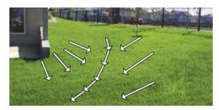
Internal drainage swales (above and below).
