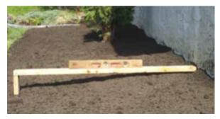
Dirt or sod should slope down from the wall on a continuous angle.
