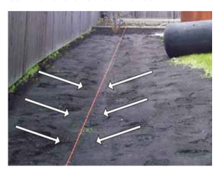
A swale should slope to channel water away from the home.
