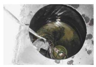
A sump pit with submersible sump pump.
