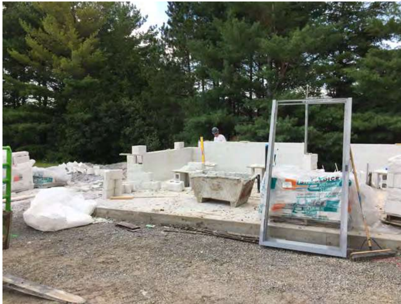
Image 3: Building Wall Block Installation
