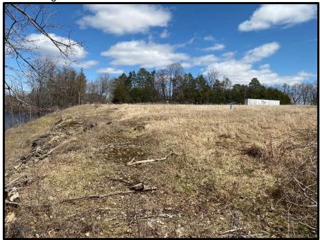
Photo 2: Photograph taken from top of slope looking to the north. Area of slope observed to be generally covered with mature vegetation such as bush, trees and grass. No signs of active erosion observed.
