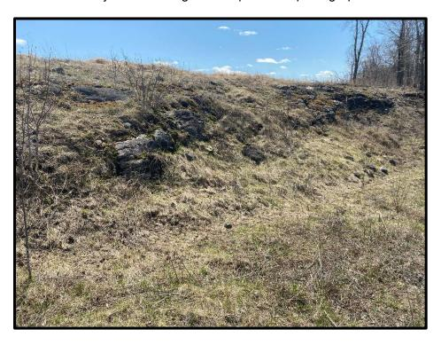
Photo 5: Photo of slope taken from top of slope. Slope observed to be covered with mature vegetation. No signs of active erosion observed
